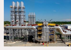
Alfa Laval is a provider of optimum solutions for high-performance waste heat recovery. The Alfa Laval Aalborg AV-6N is able to recover waste heat from various exhaust gas sources. It increases the total efficiency of your CCP (Combined Cycle Plant), CHP (Combined Heat and Power) or industrial plant.
