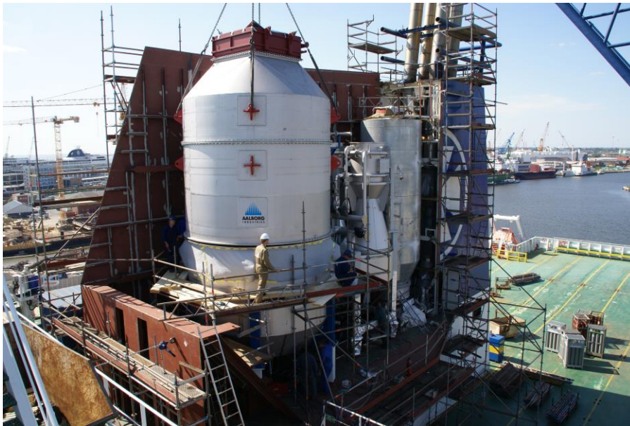
Image name PureSOx_Ficaria_Seaways_Installation.jpg
