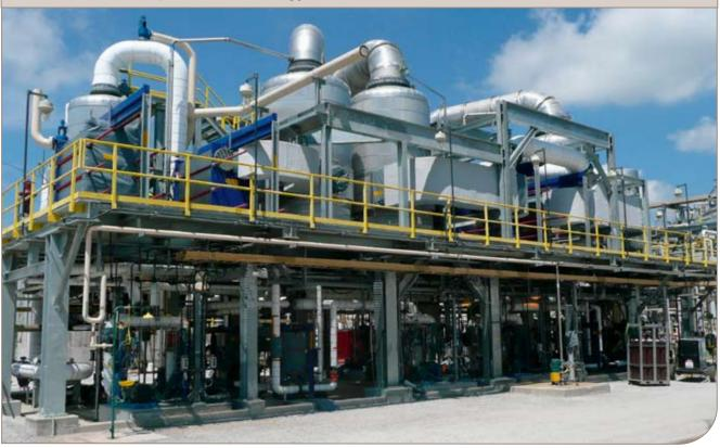
Probably the world's most energy efficient caustic soda evaporation plant at Olin in Baton Rouge, USA. It is the largest caustic soda plate evaporation plant in the world with a capacity of 1,100 tpd. Today Alfa Laval has the capability to design and build plants with capacities of up to 2,000 tpd, covering all market requirements.
