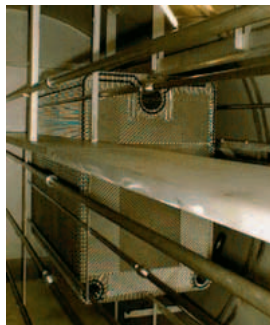
The Alfa Laval plate desalination heat transfer area in Titanium Grade 1
