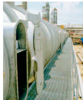
The Alfa Laval plate desalination heat transfer area in Titanium Grade 1
