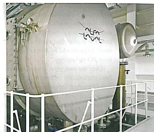
Two Alfa Laval high efficiency evaporators, type MEP-6-900, have been installed on board Norwegian Breakaway. These are each capable of producing 900m 3 per day
