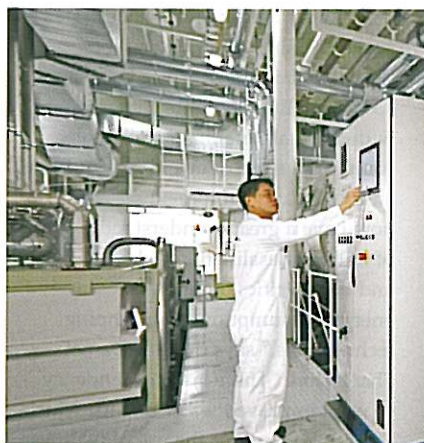
Two Alfa Laval high efficiency evaporators, type MEP-6-900, have been installed on board Norwegian Breakaway. These are each capable of producing 900m 3 per day
