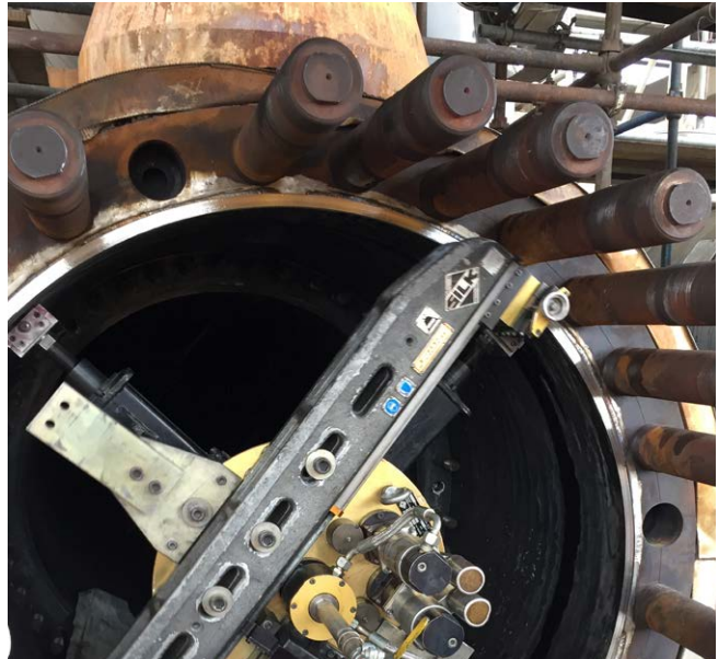
Machining of gasket surfaces using a custom-built boring machine.
