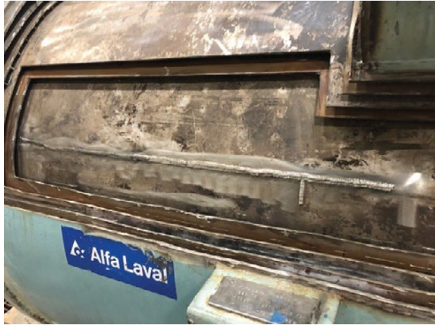
Spiral window repair cutting down to root of problem.
