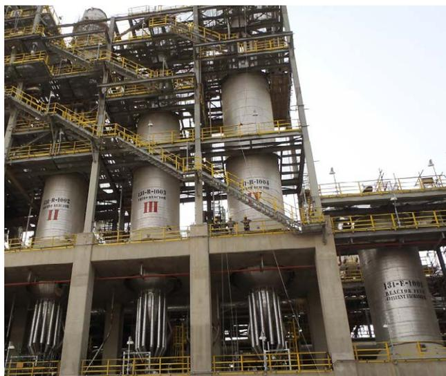
Alfa Laval Packinox combined feed/effluent heat exchanger installed in a refinery.
