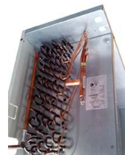
T-connection for hot-gas ready
