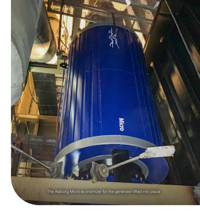
external steam space, for example by sharing the steam drum of a connected oil-fired boiler, it has no steam space of its own. This makes it small and extremely light.
