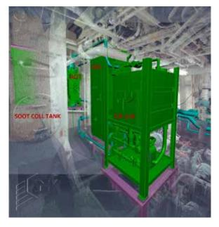
This pre-engineering visualization offers an opportunity to evaluate the suggested installation and determine how the piping should be routed, as well as the need for support of the components.
