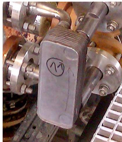
Alfa Laval tantalum heat exchanger installed at United Initiators.
