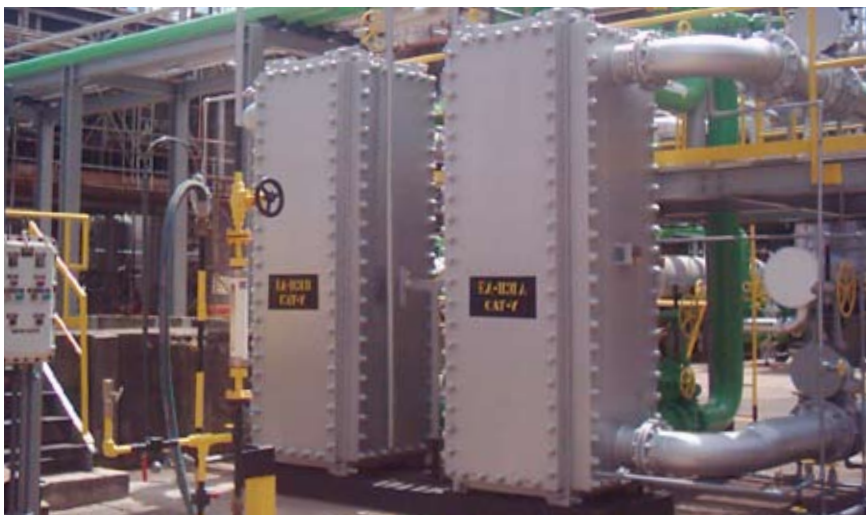
The two space- and maintenance-saving Compablocs at the Braskem plant
