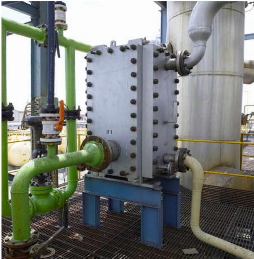
in its plants. The heat exchangers are used as condensers, reboilers, vaporizers and coolers.
