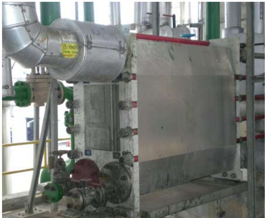
In the Alfa Laval double-wall plate heat exchanger there is no risk of intermixing between the cooling water and the product (MDI).
