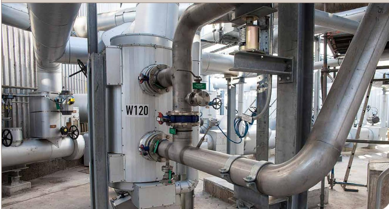
High resistance to material fatigue, outstanding thermal efficiency, minimal fouling and a well-developed service network were the major reasons for Rütgers to install two Alfa Laval DuroShell plate-and-shell heat exchangers in its coal tar oil depot in Castrop-Rauxel, Germany. “The DuroShell heat exchangers fulfilled our expectations entirely, right from day one,” says Dietmar Scholl, operations technical officer at the Rütgers Group.
