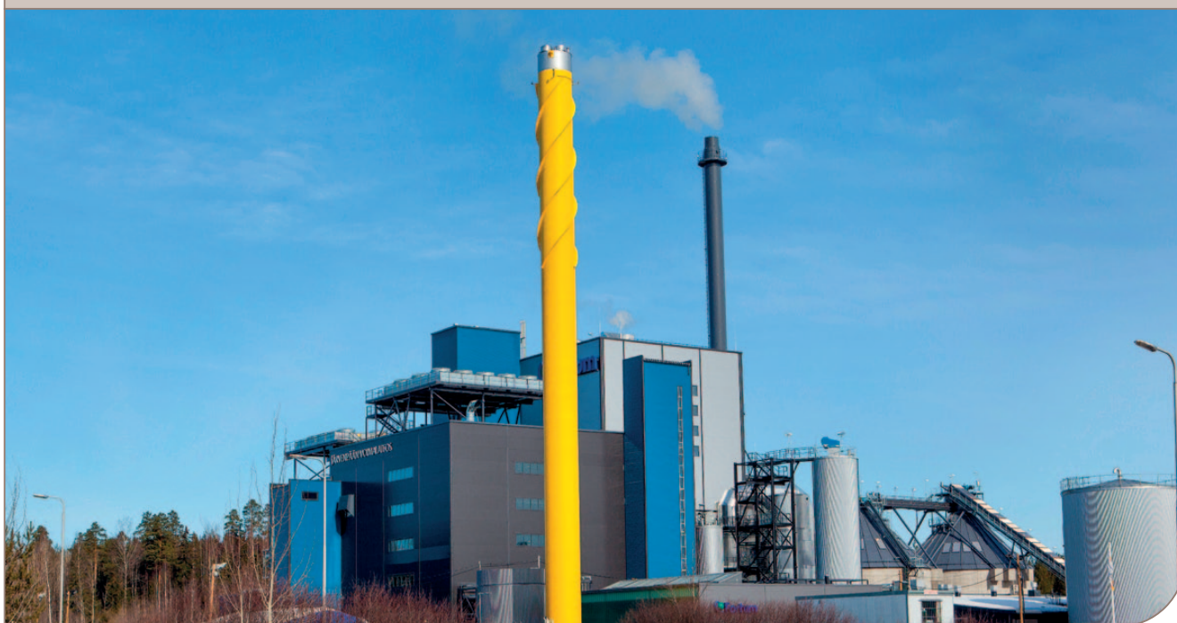
Biofuel-fired CHP plant at Järvenpää, Finland
