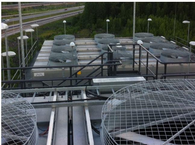
Alfa Laval FBLGS-1200-20-3A10 closed-loop coolers
