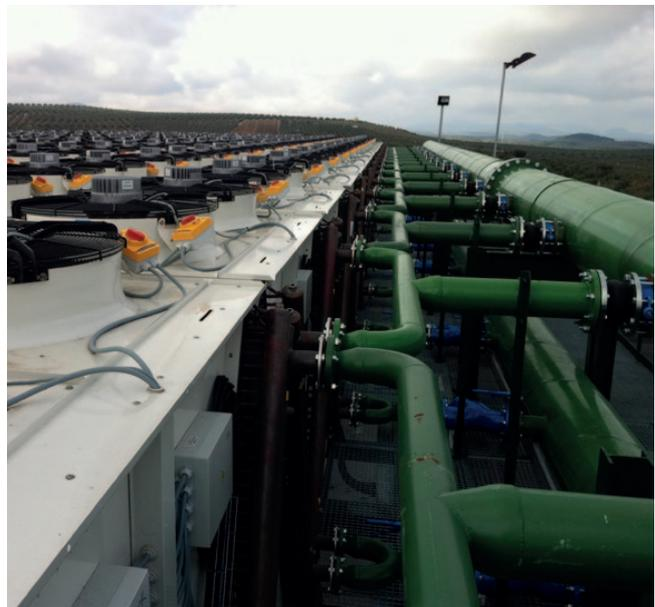
Collectors and electronic motors of the Air Heat Exchangers in detail while working. Each fan motor is provided with a safety switch to allow its manual shut down.
