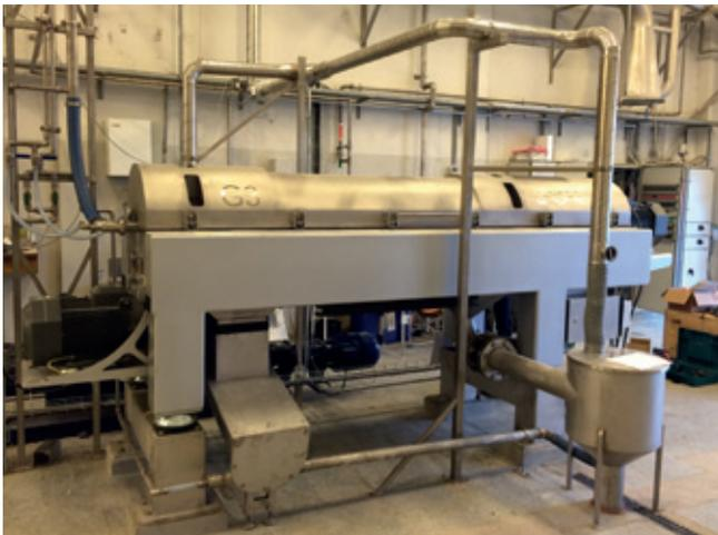
The new fully automatic Alfa Laval ALDEC G3-75 decanter at the Vejen Wastewater Treatment Facility dewateres biological wastewater sludge up to a dry solids content of nearly 24%, a clear improvement over the 16-18% that was possible with the old belt press.
