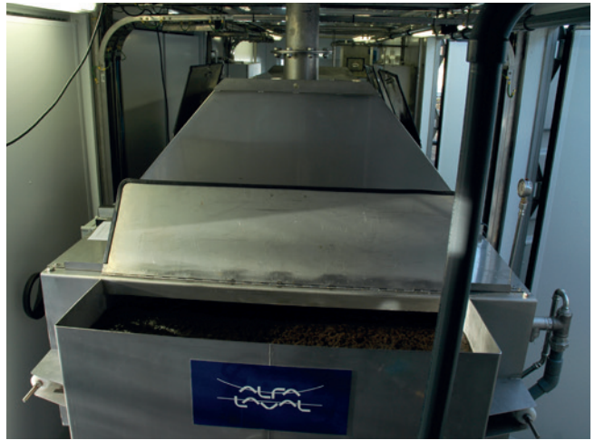
The containerized Alfa Laval AS-H Belt Thickener at Ruhrverband's Arnsberg-Wildshausen wastewater treatment plant.
