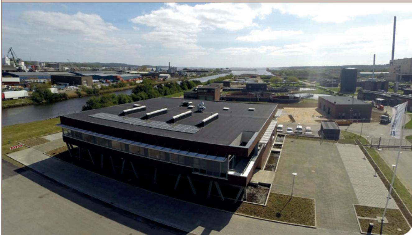
**The Danish municipal wastewater treatment plant Horsens Vand A/S has for its central treatment plant invested in a new Alfa Laval ALDEC G3 decanter, which increases the dry solids content in sludge for disposal by 4-6%. This gives an annual saving of EUR 100,000 – 130,000 on the costs for disposal of sludge.**
