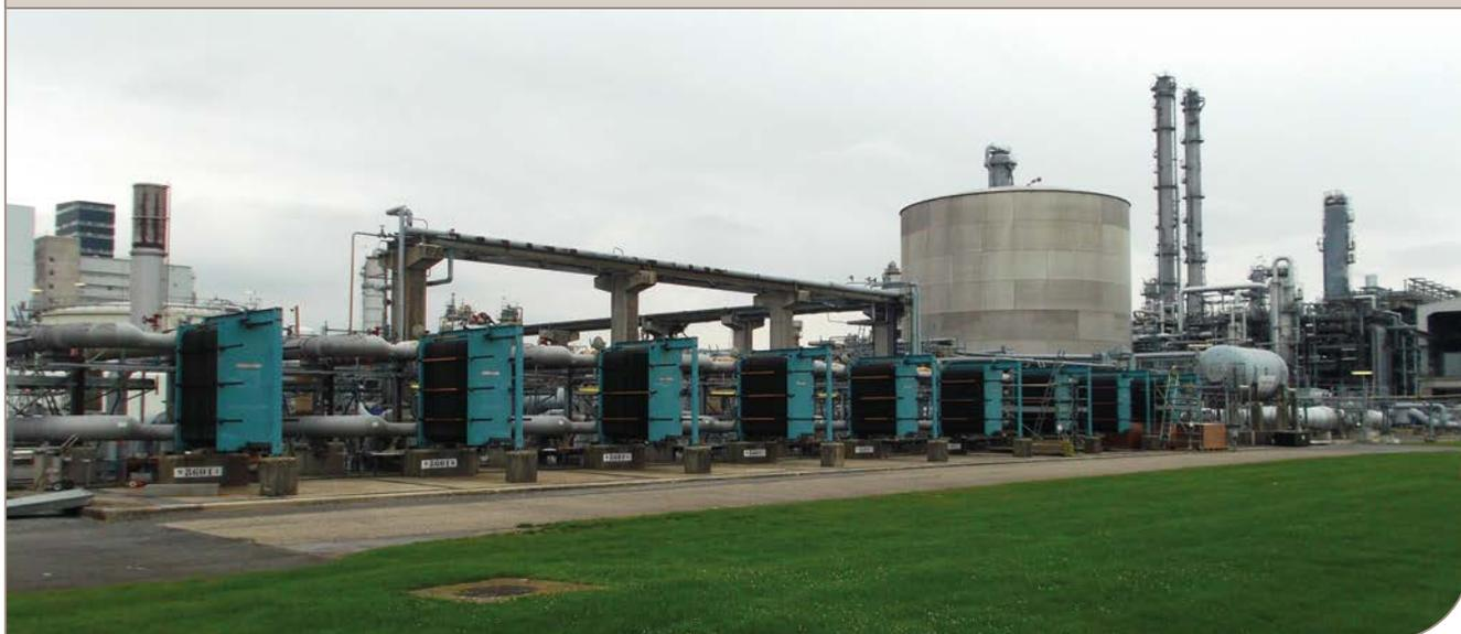
Nine Alfa Laval M30 units are responsible for cooling down the process water of the steam cracker.
