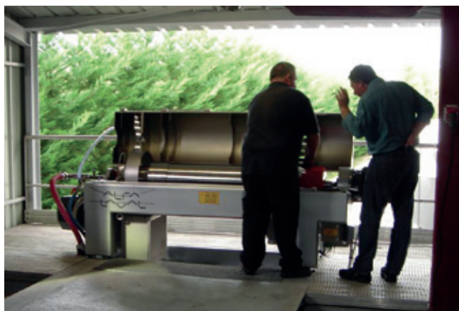
Installation of the Foodec decanter at Rabastens
