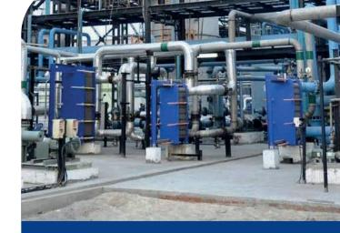
The Tuticorin Alkali Chemicals and Fertilizers Limited plant uses six medium-sized Alfa Laval Gasketed Plate Heat exchangers, in the following positions:
