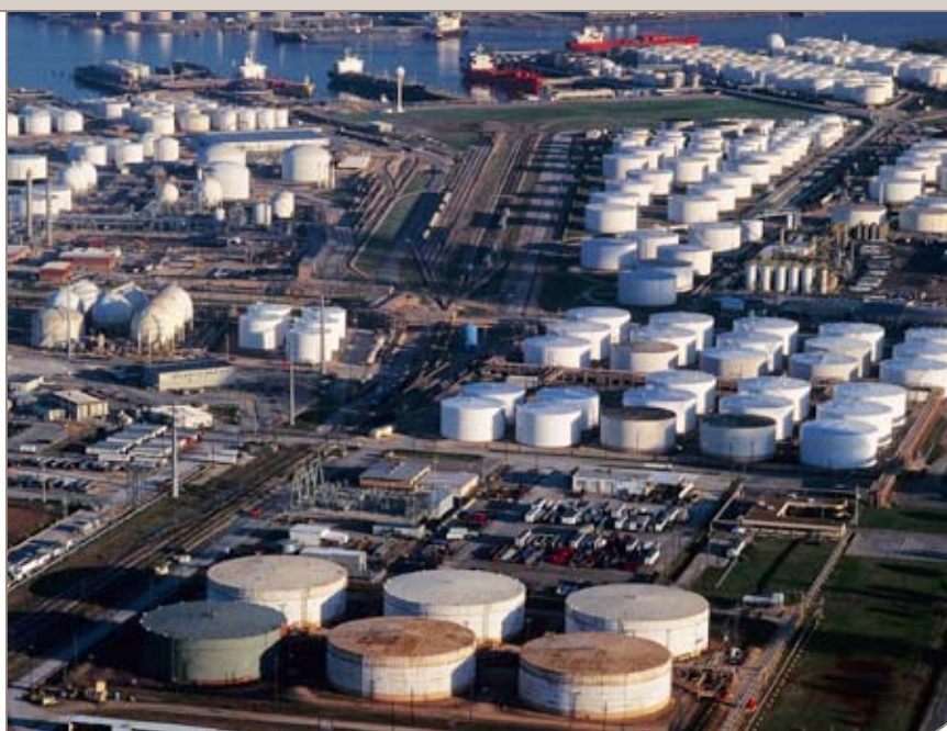
Tank terminals require efficient pumping solutions for unloading and loading products of varying qualities, in all temperatures. The customer, a molasses transshipment company in Odessa (not shown) found Alfa Laval Rotary Lobe Pumps to be the most cost-effective solution.
