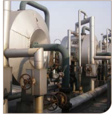
The single-channel technology, spiral shape and hinged door make the Alfa Laval spirals long-lasting and easy to maintain.
