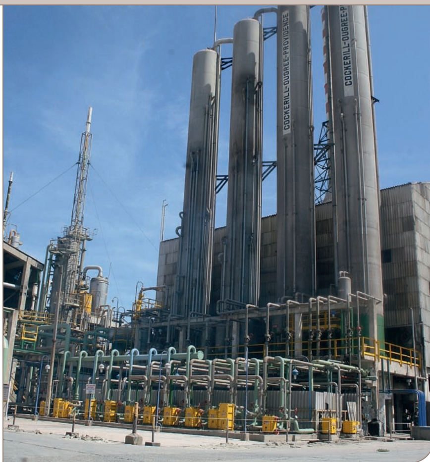
Thirteen Compablocs used as nitric acid coolers at the Monómeros Nitric acid plant in Colombia.
