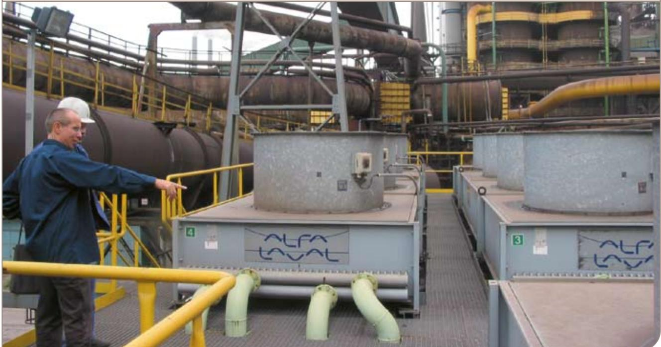
Alfa Laval air coolers have now replaced an open cooling tower water system at Mittal Steel Ostrava.
