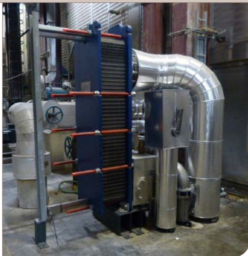
The AlfaCond 400 condenser at work in the Sappi Maastricht mill.
