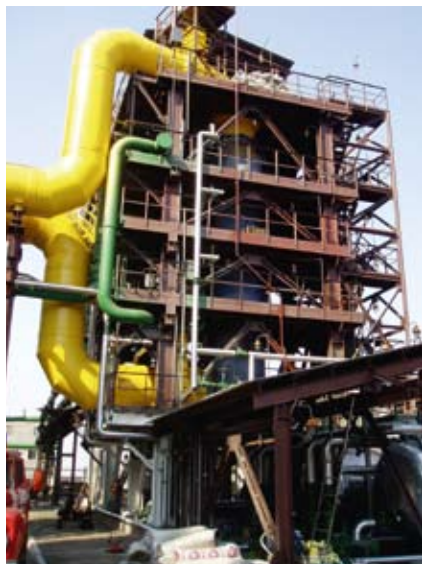
Final coke oven gas cooler. An Alfa Laval spiral column installed at Avdeevskiy coke processing works.
