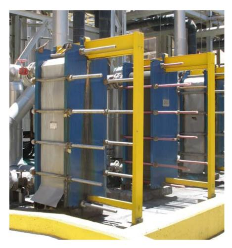
is carried out on one of the 16 heat exchangers each year. The units are designed to make physical maintenance as straightforward as possible. The plates hang on carrying bars, making it easy to open the bolts and clean when necessary.
