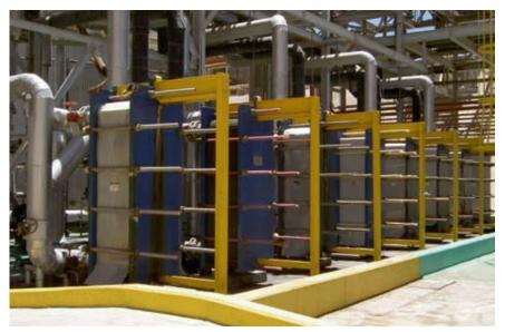
Six of the 16 heat exchangers at the Barrick Zaldivar copper mines in Chile. The mechanical construction of the Alfa Laval Plate heat exchangers makes them easy to open and clean by unscrewing the tightening bolts.
