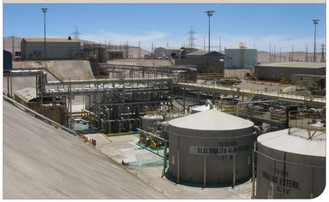
A view of the facilities at the Barrick Zaldivar copper mines in Chile. Eight of the 16 heat exchangers are visible in the middle of the picture just behind the small tank.
