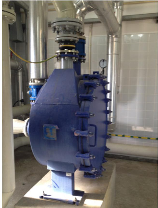
Prosna uses their two Alfa Laval Spiral Heat Exchangers for digester heating.
