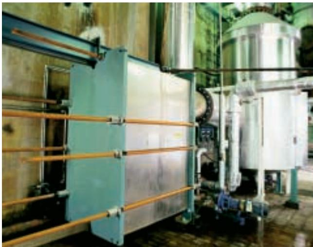
The plate evaporator installed as a replacement for a shell-and-tube evaporator at Kemira AB in Helsingborg, Sweden.
