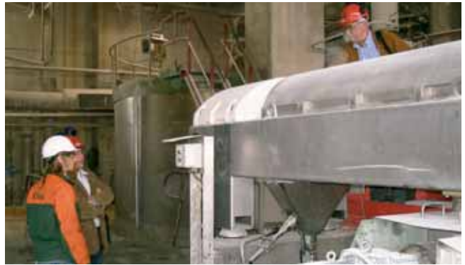
"The decanter centrifuge takes up only 20% of the space required for a vacuum filter," explains Pål Salberg – project engineer at Södra Cell Tofte – to Thomas Svensson, sales engineer at Alfa Laval Nordic.
