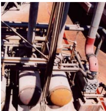
The Compabloc replaced a shell and tube unit on a quarter of the footprint.
