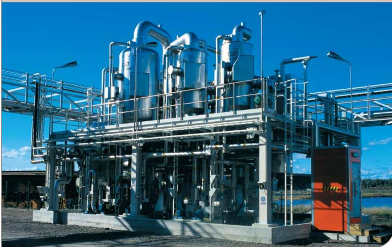
When Akzo Nobel invested in a new plant to concentrate caustic soda, it decided in favor of a solution with plate evaporators resulting in substantial savings in installation and maintenance costs.
