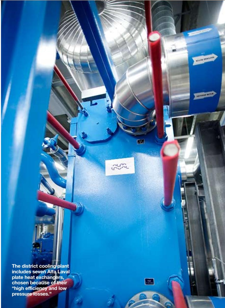
The district cooling plant includes seven Alfa Laval plate heat exchangers, chosen because of their “high efficiency and low pressure losses.”
