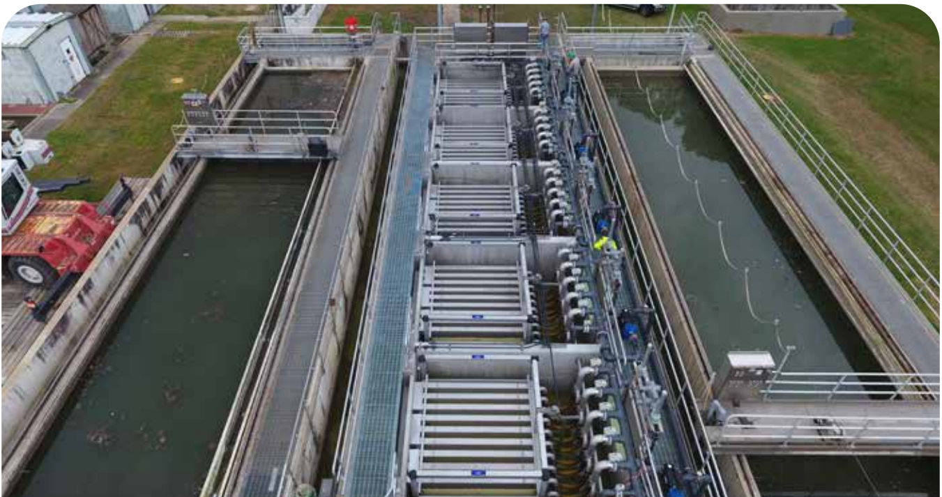
Alfa Laval AS-H Iso-Disc retrofit installed in an existing traveling bridge basin
