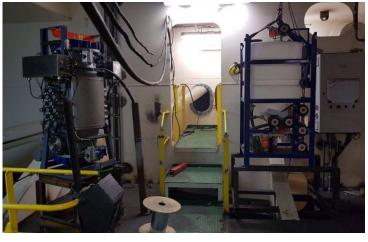
Air filter (V201-8) installed upside down.
