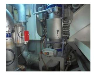
CIP unit installed on a higher level than UVR.
