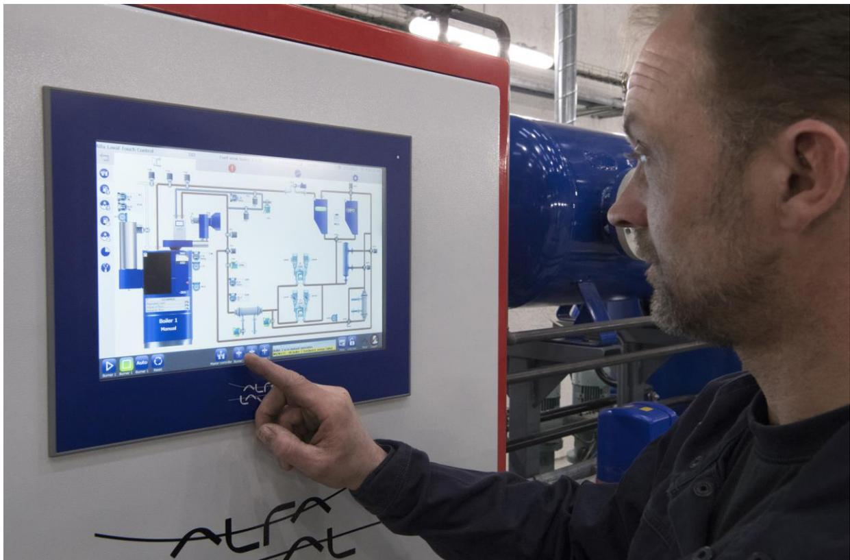
With its graphical touchscreen display and intuitive two-touch navigation, Alfa Laval Touch Control is a major leap forward in boiler control technology. As the new common control platform for all Alfa Laval Aalborg boilers, the system will be a familiar interface for crews, regardless which boiler they work with. Already it can be found aboard a range of newbuilds, and additional deliveries are underway.
