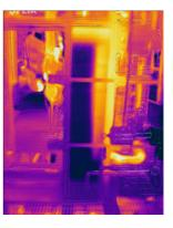
Lower velocities, less turbulance, faster fouling and less performance in a district heating application.
