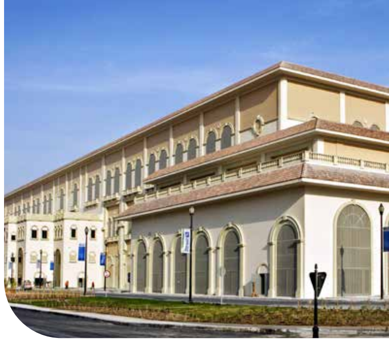
The building accomodating the cooling plant has an architecture brought into harmony with the surrounding buildings.
