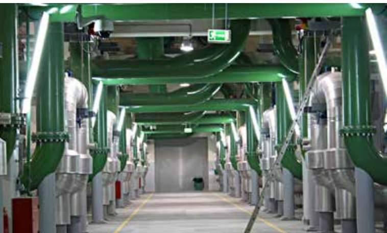
From the cooling plant, a pipe network provides the cooling for all the amenities – residential, commercial and sportive – for the entire manmade island of The Pearl Qatar.
