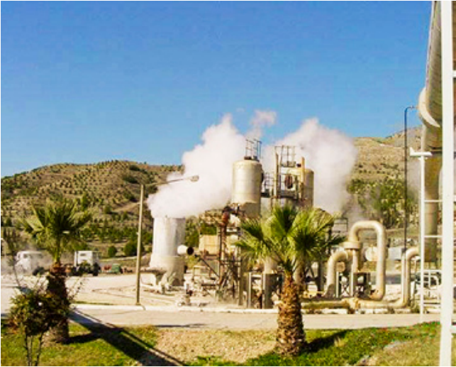
The Balcova project is an interesting “model project” distributing heat and domestic tap water to local households via a district heating network and with geothermal water as medium.
