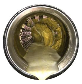
Blockage of outlet line caused by floating solids leaving the tank last
