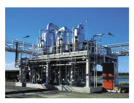
A three-effect system that evaporates NaOH from 32 to 50% at Akzo Nobel in Sweden. The system was built by the contractor Chematur Ecoplanning, using AlfaVap and AlfaCond. The need for exotic materials such as nickel makes the AlfaVap exceptionally economical in this application.
