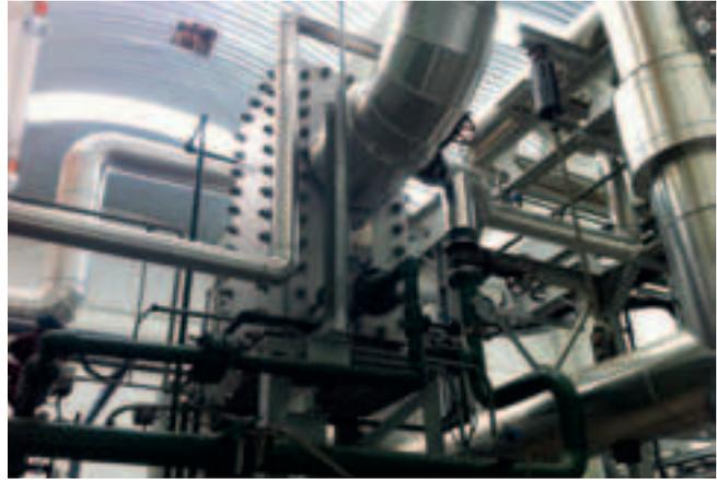
In the Miajadas plant, the main duty of these Compabloc units is to use extraction steam from the turbine to heat the boiler water from 50°C to 80–90°C. According to Rafael Godoy, "This equipment, which has been designed specifically to suit our needs, provides outstanding performance as well as being very compact." This space-saving design then made it possible to mount this pre-heater unit in the most convenient place.
