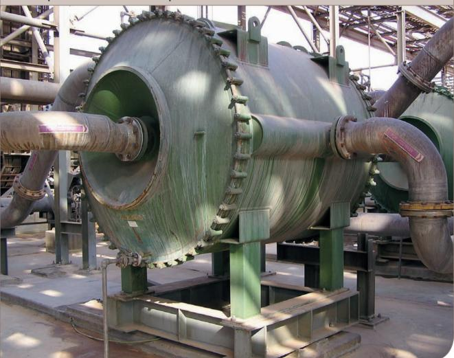
A spiral heat exchanger has two concentric, countercurrent spiral channels, one for each fluid. The curving channels provide extremely efficient heat transfer and good flow conditions for a wide variety of fluids. The design is particularly suitable for use with fouling,
