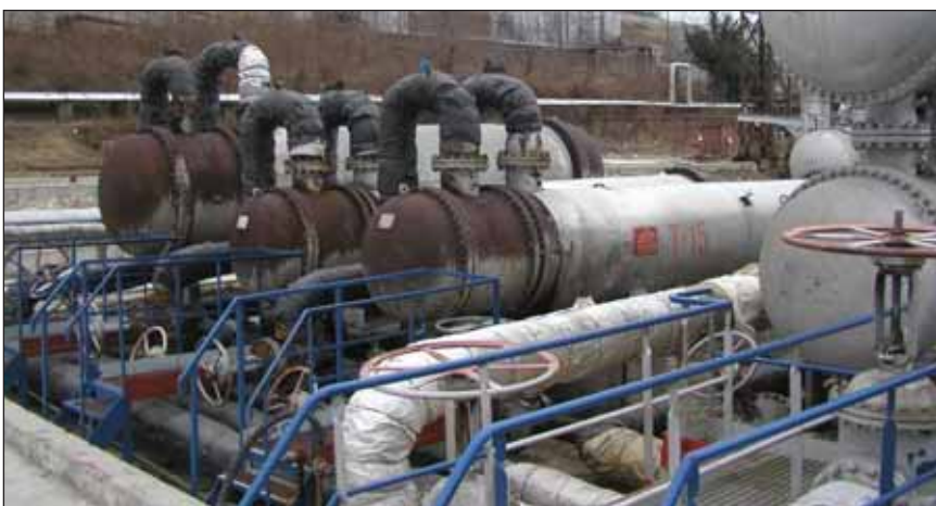
Figure 3 Difference in heat-transfer area and ground space for a S&T compared with a CPHE installation in a heat-recovery installation (atmospheric residue: 288 → 162°C; crude: 107 → 201°C; heat load: 7MW). S&T total heat transfer area is more than 1000 m 2 and CPHE heat transfer area area is only 170 m 2
