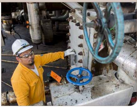
Petronas' Kerteh refinery in Malaysia has enhanced its energy efficiency by using Compabloc technology.
